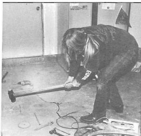
Crushin' the concrete square.
